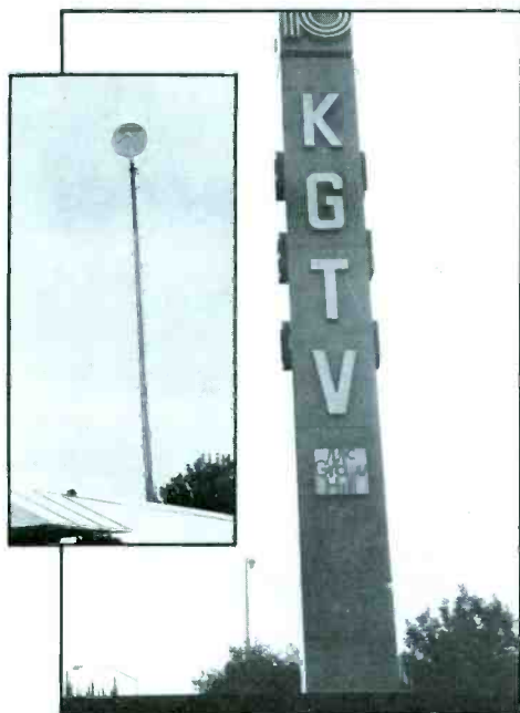
KGTV's new steerable Miniscan is installed at the station for ENG pickup.
